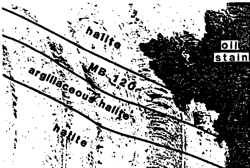
Figure 17.--Left rib of 16-L drift as in figure 16. Base of MB 120 is slightly below the center of photo, top of MB 120 is near upper left corner. Dark portion of picture to right is oil stain. Pipe about 5 m (16 ft) to right.
